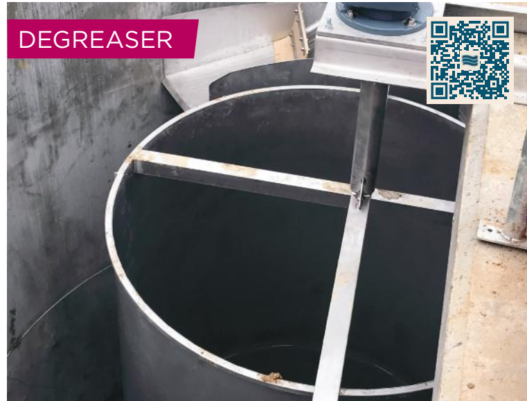
GRIT AND GREASE REMOVAL SYSTEM
