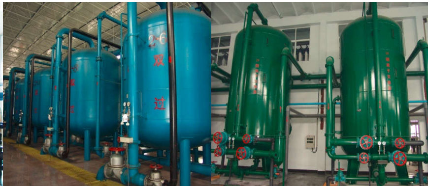
Sand filter exchanger
