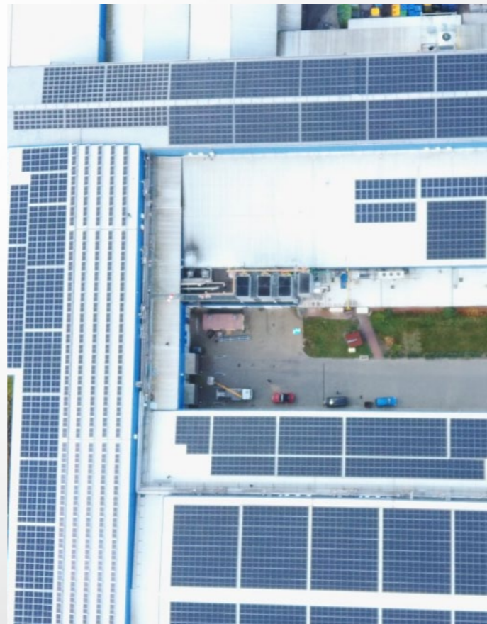
1.5MW PV Rooftop Project in Poland
