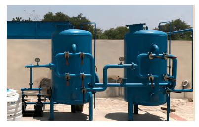
Activated Carbon Filter (ACF) works on the principle of adsorption. The filter media adsorbs or reacts with pollutant molecules, and then filtered water is drained out.Activated carbon which is used as a medium to remove contaminants is a natural material derived from coconut shells, lignite, bituminous coal, etc. Activated Carbon Filters are installed after MGSF to remove
