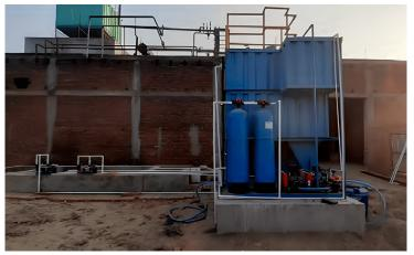
UY Trienviro designs, fabricates, installs and commissions different capacities of packaged sewage treatment plants as per the customer's requirements. These are suitable for rural areas, highway rest stops, hotels, restaurants and hospitals mainly where population is small or space is less or required plant capacity is small. The treatment scheme starts from bar
